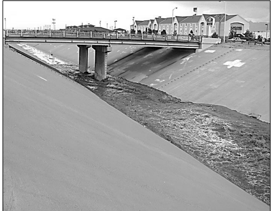
FIGURE 7. Storm surge within a concrete flood control channel in Albuquerque, NM. Downstream the water is six inches deep, upstream it is nearly five feet deep, with the leading edge moving 20-30 mph. Photo taken June 23, 2009. Image courtesy of Albuquerque Metropolitan Arroyo Flood Control Authority.
